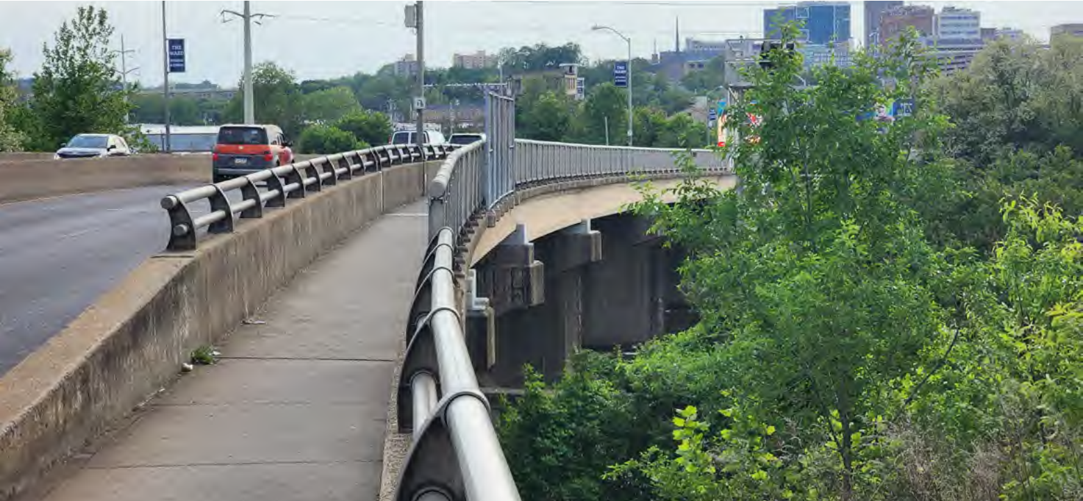
Hamilton Street Bridge over the Lehigh River
